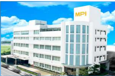
Operations Plant 2 Zhubei, Hsinchu (2012)
