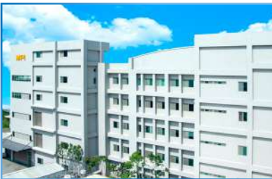
Operations Plant 3 Zhubei, Hsinchu (2021)
